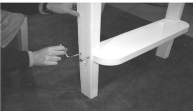
Install Foot Rest using (4) 3" Hex 1/4" Lags (Left Picture)
