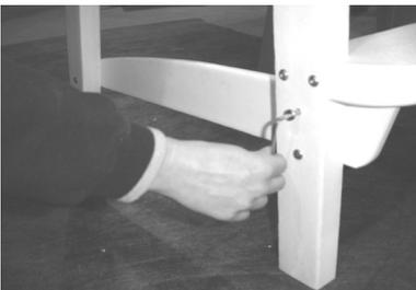
Install (2) Side Leg Stretchers using (6) 2-3/4" connector bolts. Finger tighten with flat & lock washers and nuts. Do not tighten at this time (Left Picture). Install Rear Leg Stretcher using (2) 1-3/4" Phillip's Head Screws.
